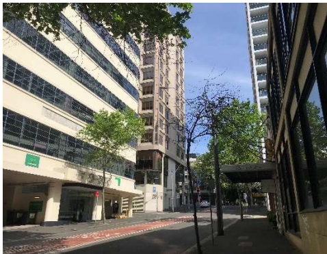
Figure 33 - View south along Riley Street towards William Street with the subject site to the RHS of image.
