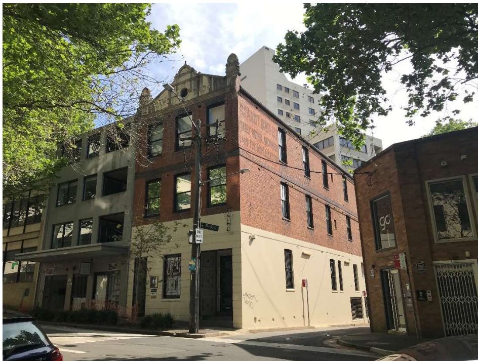
Figure 44: 41 Riley Street – 'Brandt Bros Building', on the corner of Busby Lane, Woolloomooloo.
