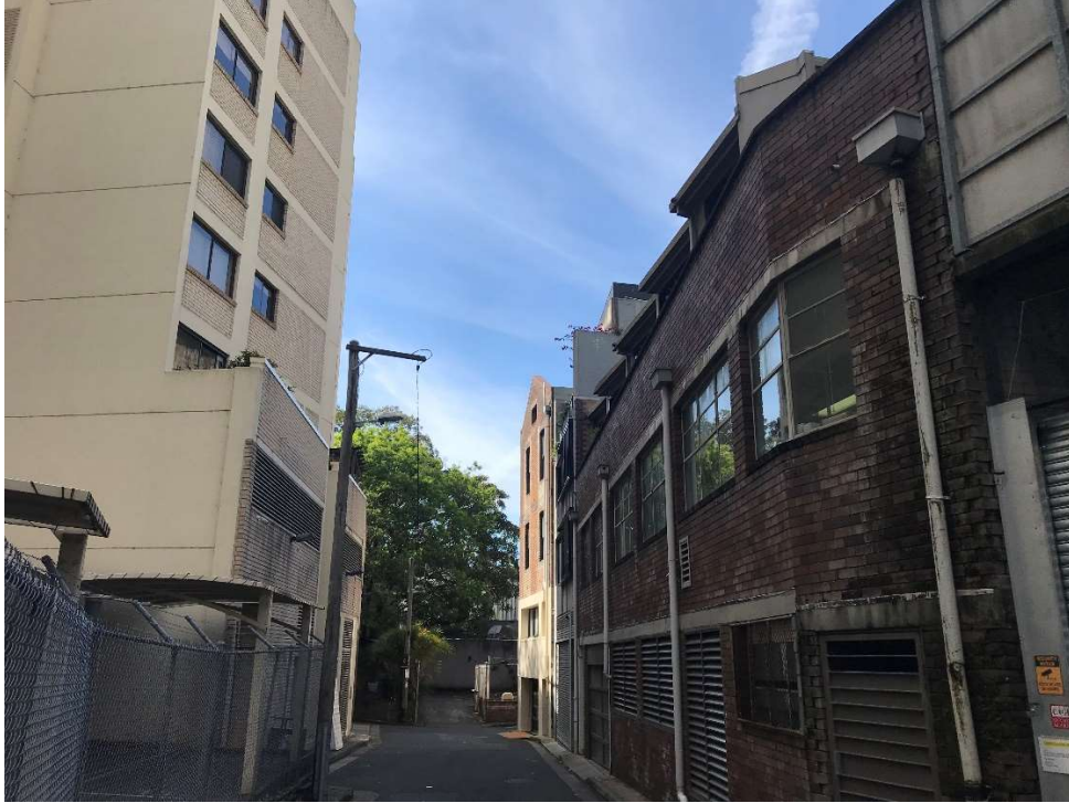
Figure 40 - Rear view of 51 Riley Street from Busby Lane. Note the proximity of the multi storey residential building immediately behind the subject site.
