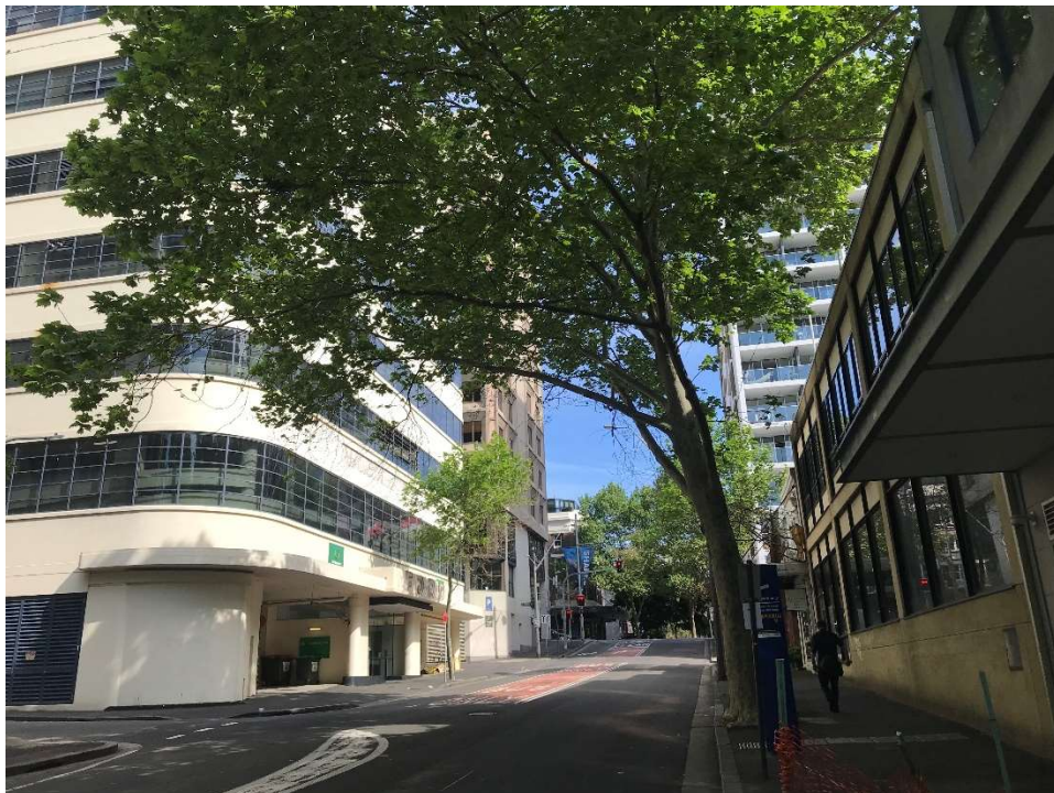
Figure 45: 46-48 Riley Street – Hastings Deering Building „ Woolloomooloo. The proximity of the subject site can be seen to the right of the image.
