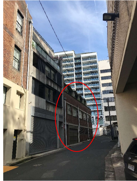
Figure 38 - View north along Busby Lane with the rear elevation circled.
