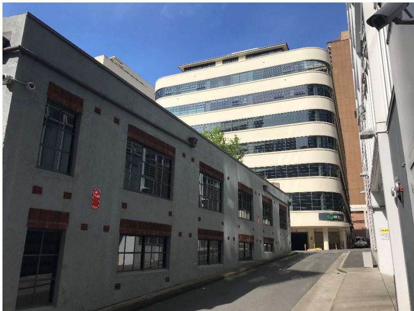
Figure 47 - View of the southern elevation of the former garage, which has now been adapted, with the Hastings Deering building beyond.
