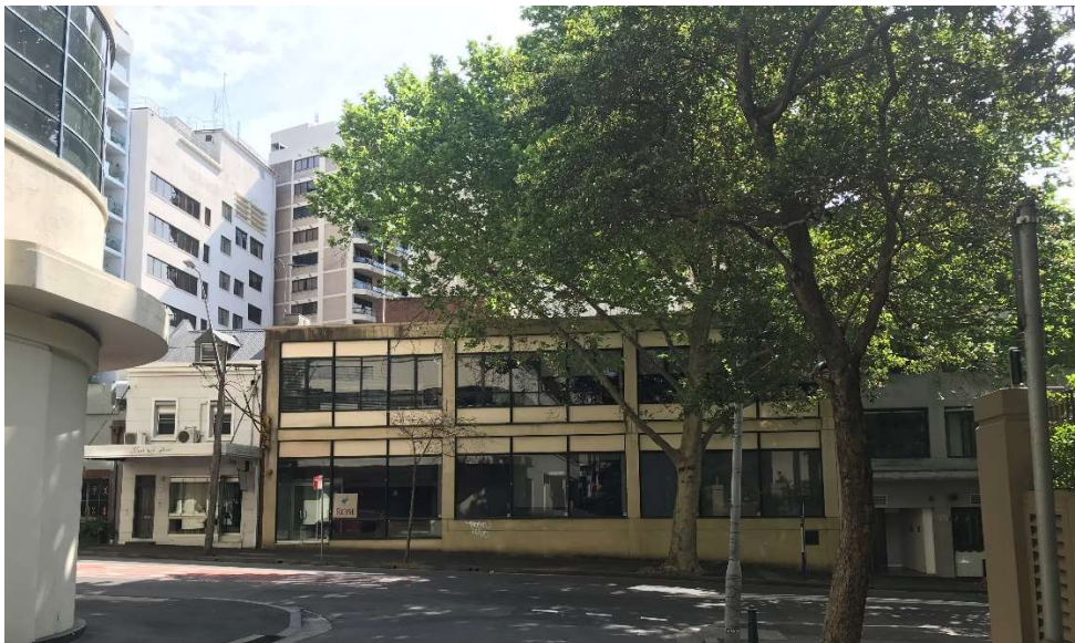
Figure 39 - Riley Street facade viewed from Kennedy Lane. The contemporary residence is to the right of the site, and the shop top style building to the left.
